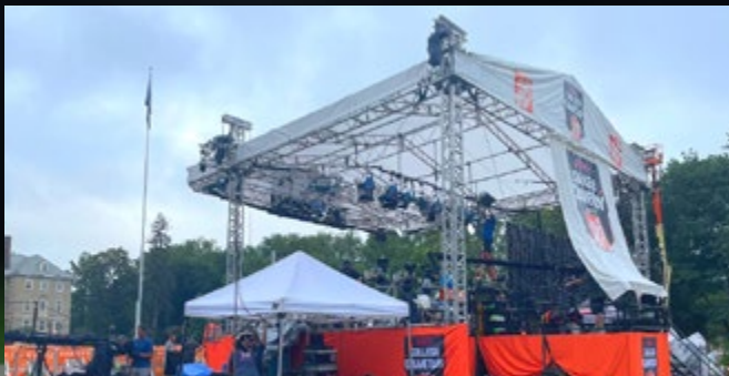
Stahl Sheaffer provided structural inspection for the ESPN Game Day Stage in University Park, PA
