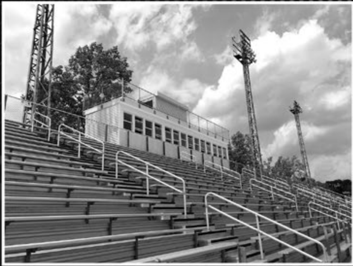
Selinsgrove Football Field Pressbox Design & Light Inspection
