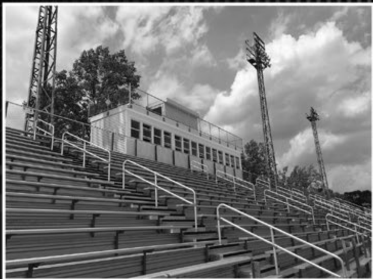
Selinsgrove Football Field Pressbox Design & Light Inspection
