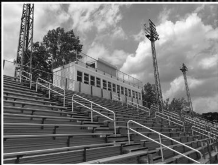
Selinsgrove Football Field Pressbox Design & Light Inspection
